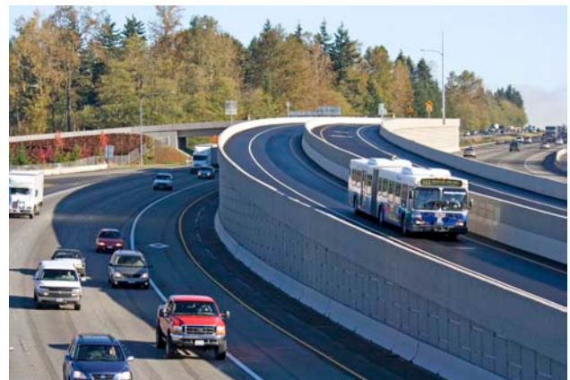
One of many bus only ramps that serve exclusive busways in the Seattle area
