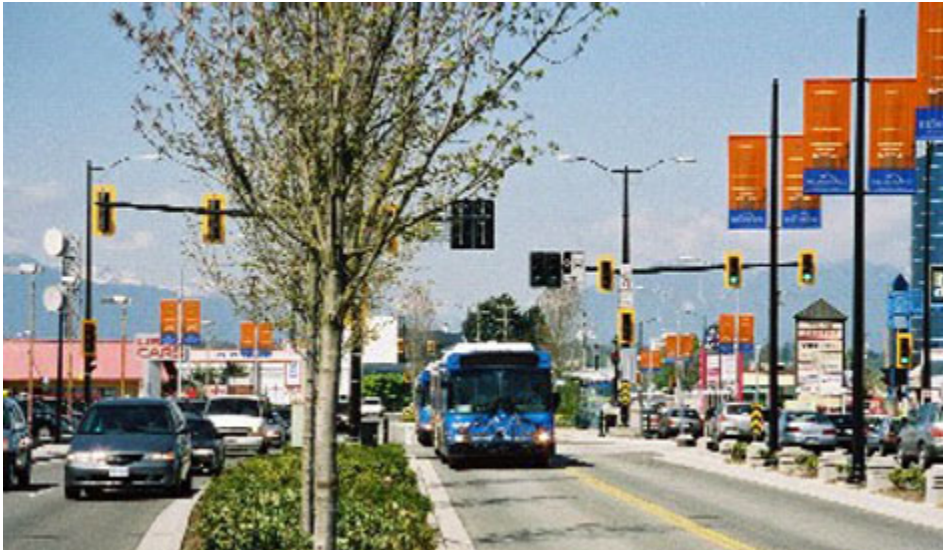
Separated running ways compete with automobiles and can bypass peak hour congestion.
