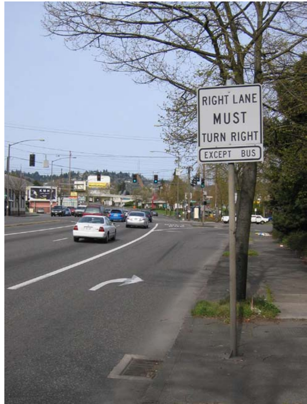
Queue jump lane along a major arterial in Portland, OR
