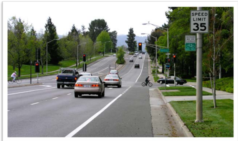
Figure 1-3: Other Principal Arterial in California
